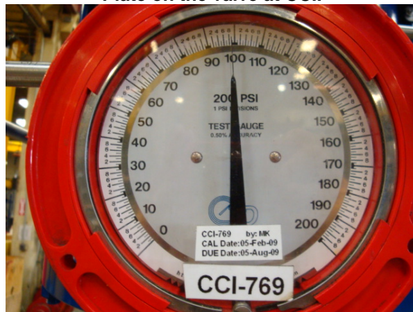
Gauge used during testing at the CCI shop.
